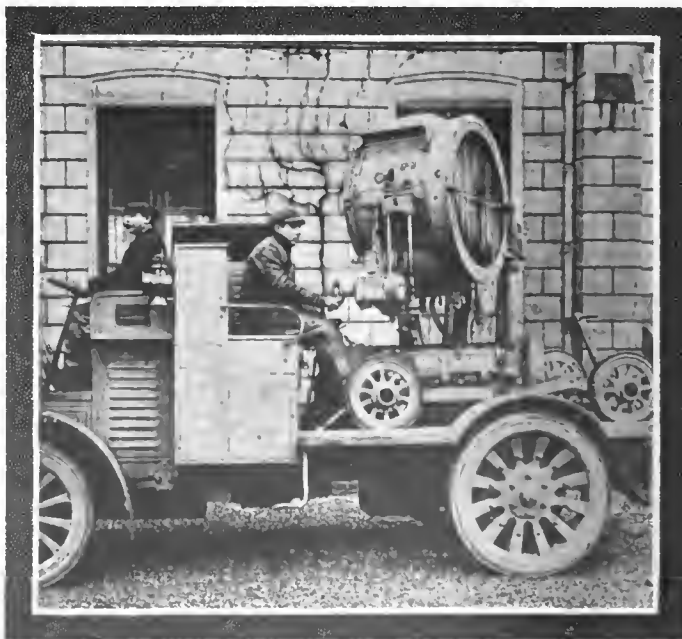
Projector raised in position for operating on the road
